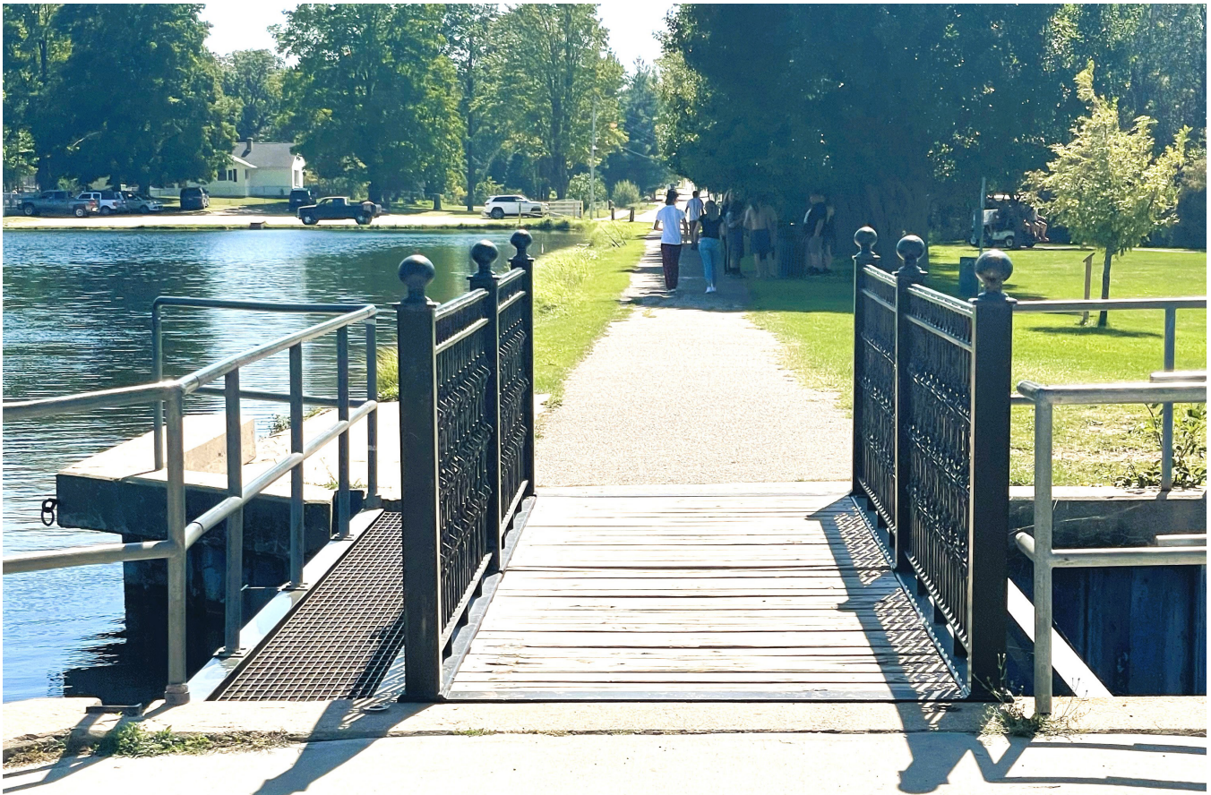
Bridge Connecting to Walkway at Lake Billings RV Park & Campground
