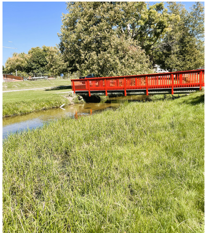
Bridge to Cross Manton Creek
